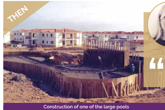
Construction of one of the large pools
