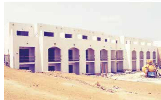
Construction continues on Boa Vista
